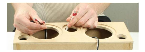
Connect the pair of white cables to the tweeter terminals.
