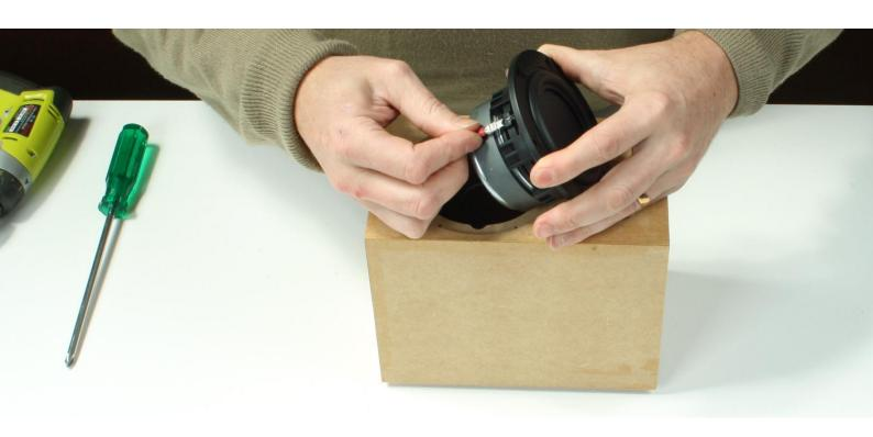
It's now time to install the driver. Push the connectors onto the driver tabs. Correct polarity is important but this is made easy by using faston connectors that are sized to avoid mistakes. The larger negative terminal goes to positive and the smaller negative goes to the other. Avoid excessive force, which can damage terminals. If you find the fit is tight, you can use a small flat head screwdriver to open them out slightly.
